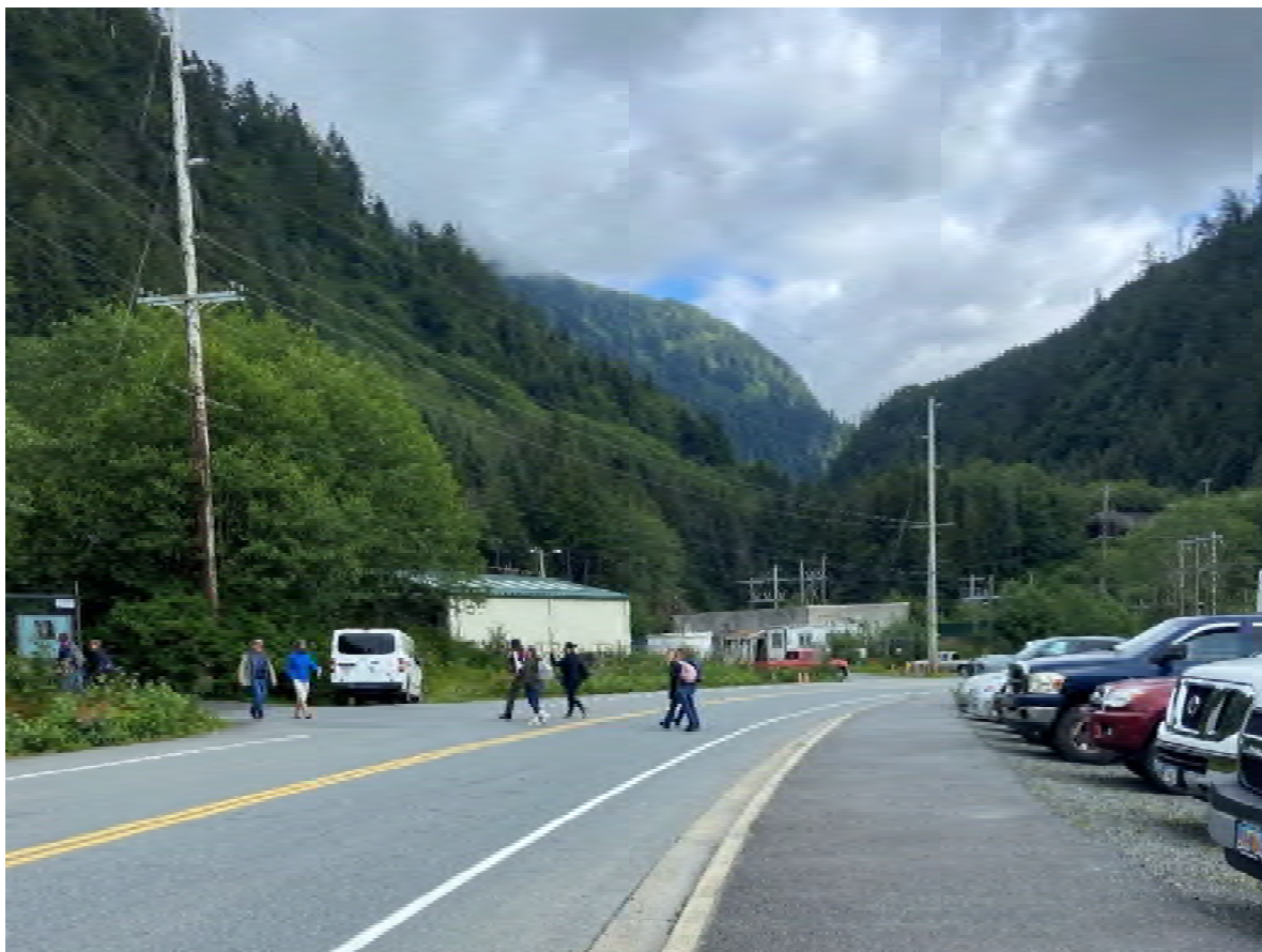
Photo 24 – Pedestrians cross Sawmill Creek Road from the Fortress parking area to the main facility
