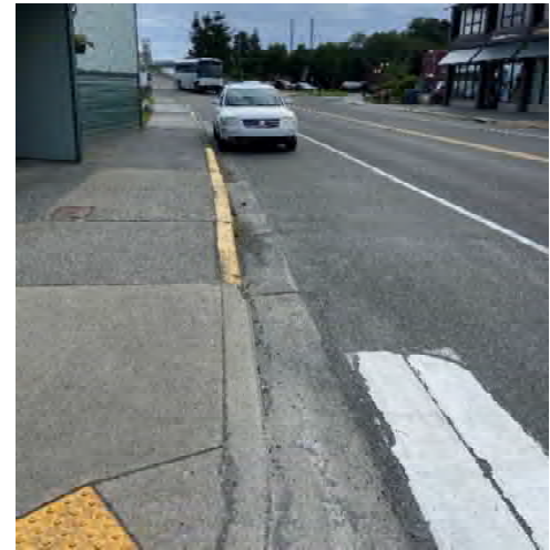
Photo 22 – Parked vehicle restricts pedestrian and approaching vehicle sight distance
